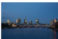
View of the Leadenhall Building in the London skyline from the West along the River Thames Copyright holder British Land/Oxford Properties Photographer Richard Bryant Photographer's email arcad@arcad.co.uk
