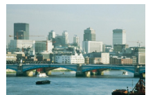
The roofscape of Lloyd's become a distinctive landmark in London's skyline in 1987 Copyright holder Arcad Photographer Richard Bryant Photographer's email arcad@arcad.co.uk
