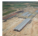
Aerial view of construction progress Copyright holder Rogers Stirk Harbour + Partners Photographer Rogers Stirk Harbour + Partners Photographer's email
