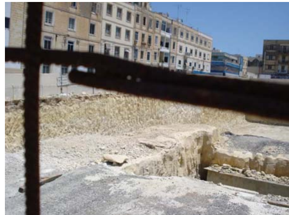
Figure 6: Excavation for the foundation of the Metropolis Tower.
