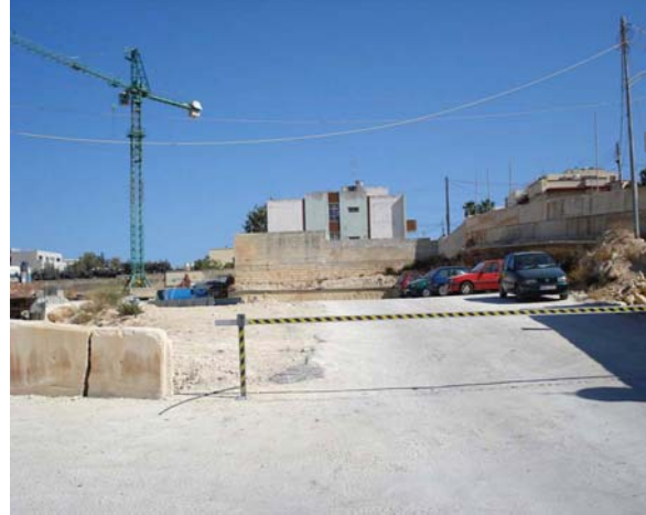
Figure 18: Pender Place construction site
